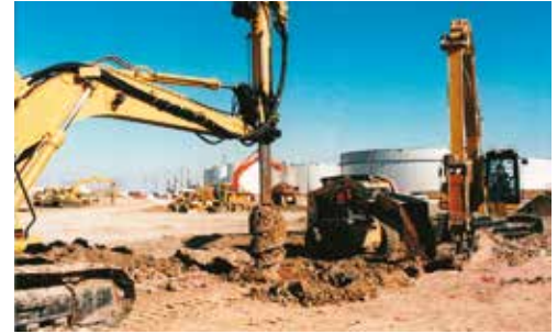
Houston Fuel Oil Terminal Company Houston, Texas
