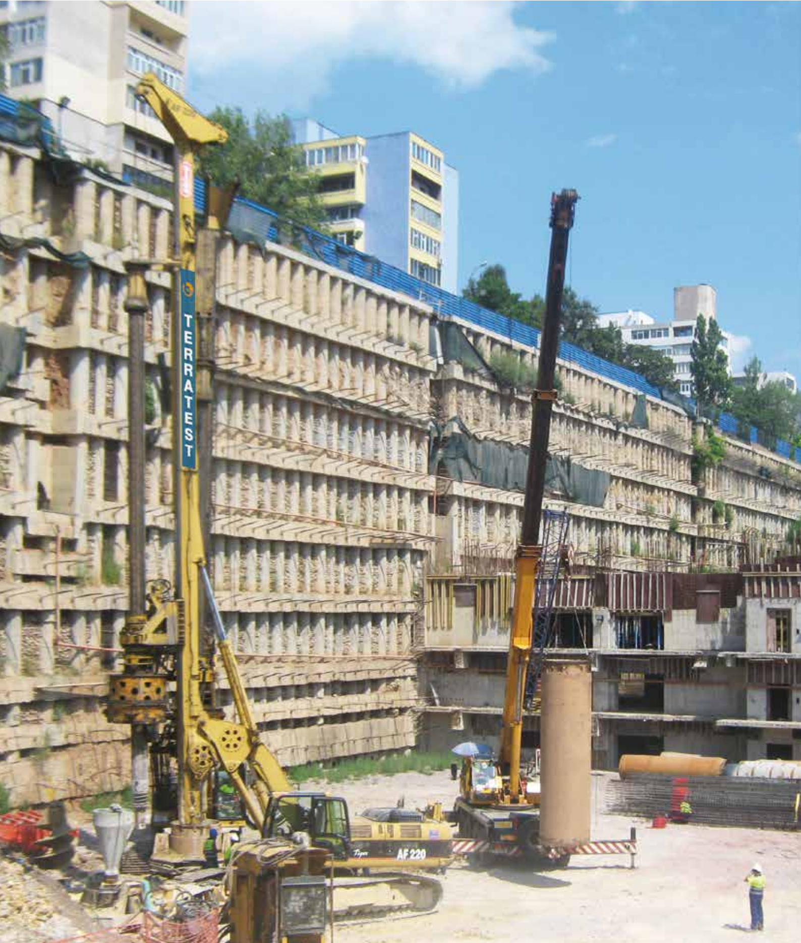
WTC Constant, Rumania Pilotes In situ
