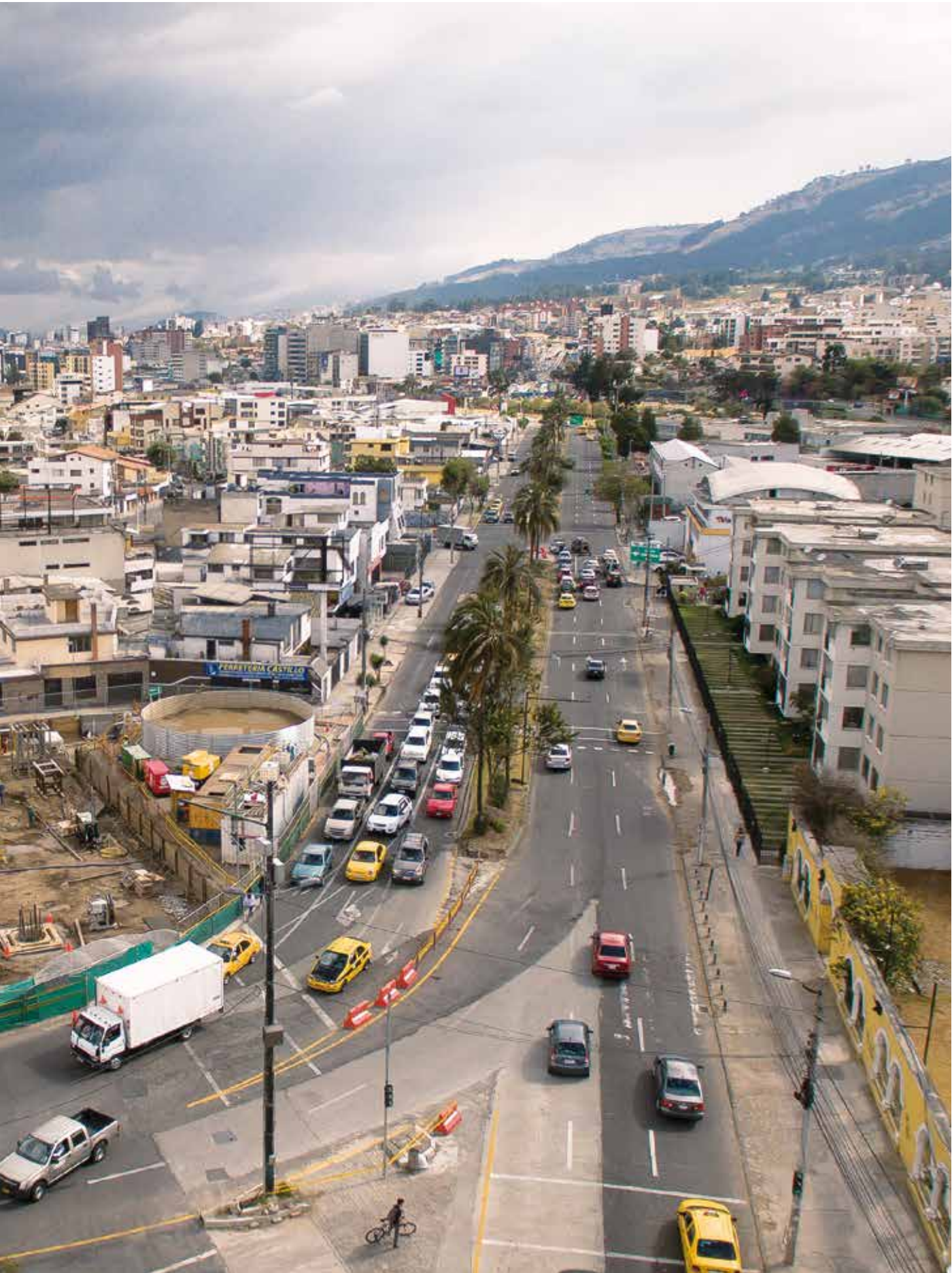
Metro Quito, Ecuador Muro Pantalla, Pilotes In situ y Jet Grouting
