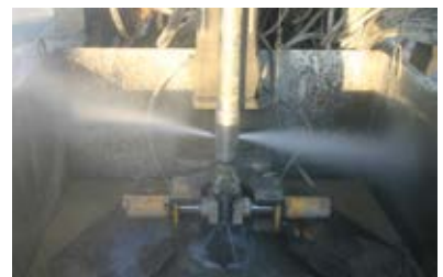
Injections de Compensation
