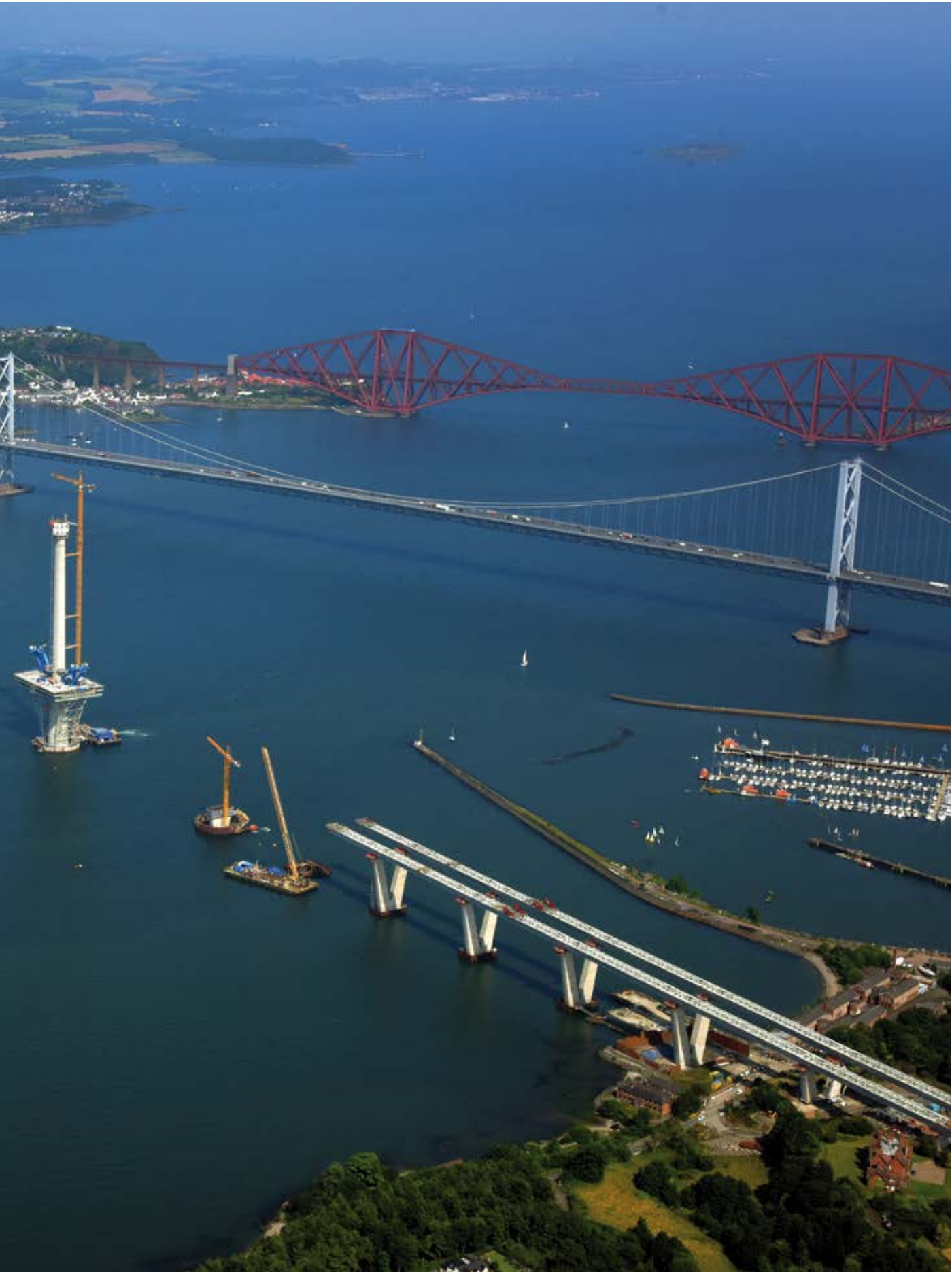
Forth Crossing Bridge. Edinburg, Scotland Off Shore Jet Grouting
